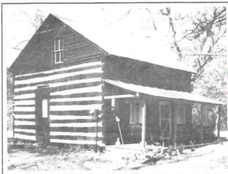
Recent Photo taken after restoration. Note the small log above the side door which could be removed to expose loopholes to shoot at the Indians. (see story in December 1994 News-Caster)
