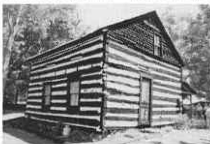
The offset logs above the doors and windows were for rifle slits. The logs were removed when needed.
