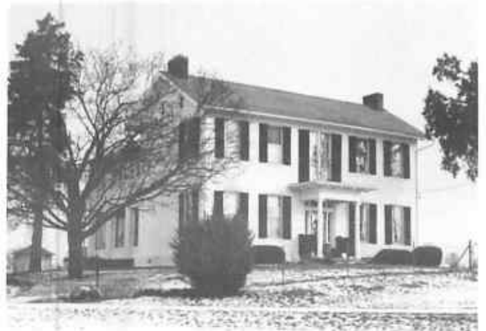
Built by Abraham Hitler, 1849, located at 6476 Tarlton Road, Circleville
