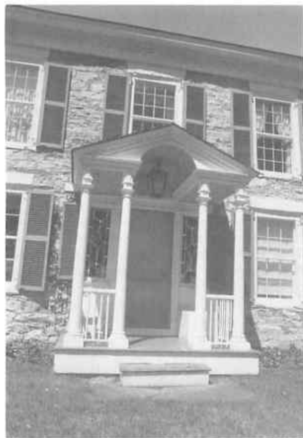
Front Porch View
