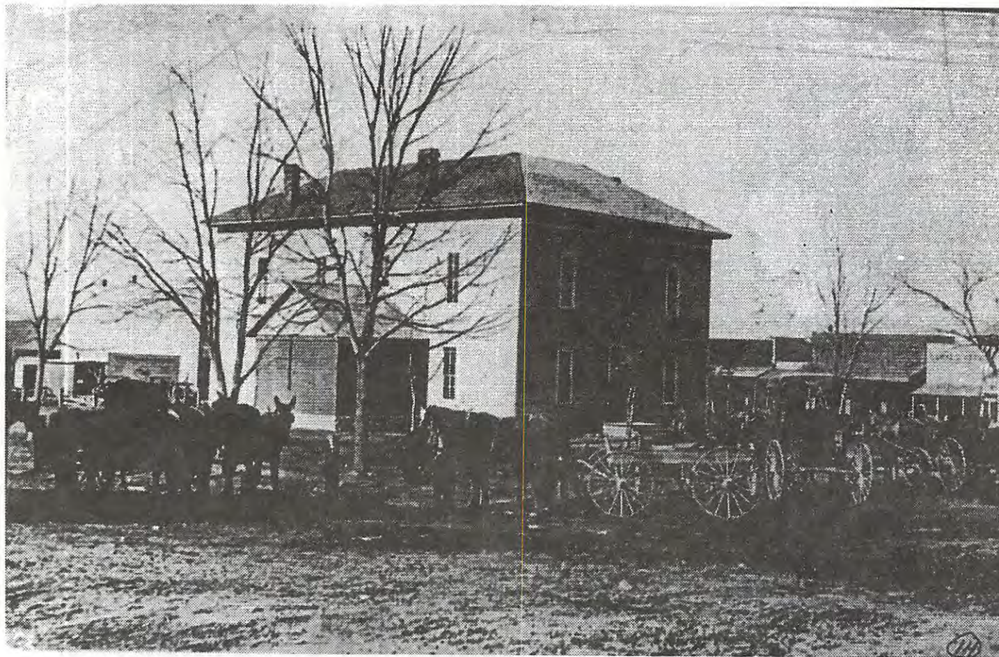
Douglas County Courthouse 1889-1937
