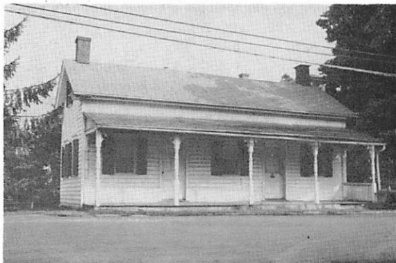
No. 135 Manor Ave.
